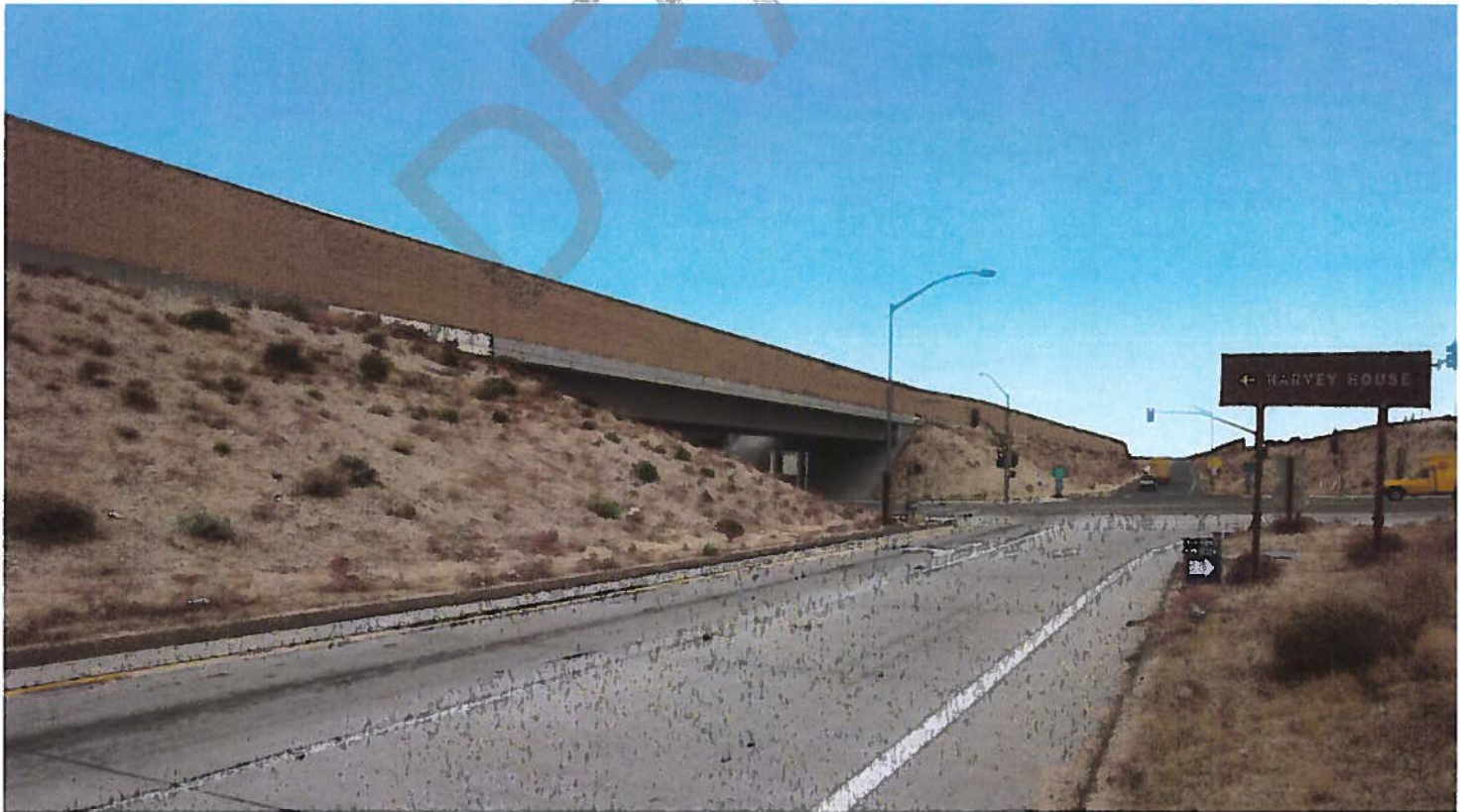
L Street Off-ramp (before)
