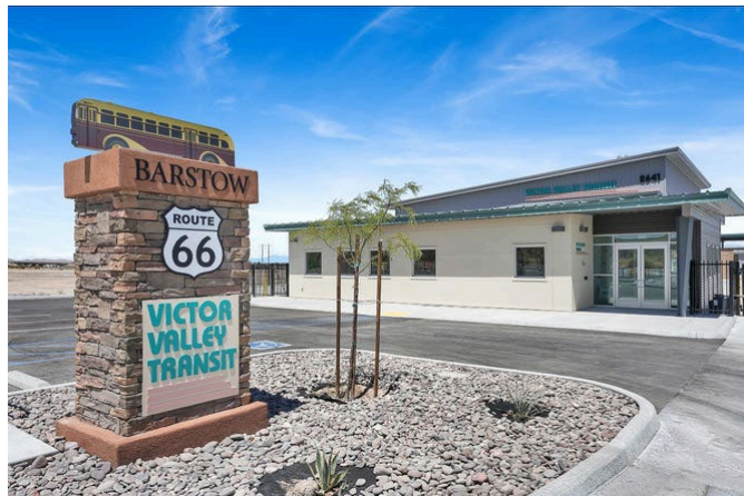
New VVTA Transit Facility
